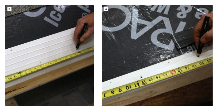
**Drip-edge nailing taken to the next level.** For regions prone to high winds, the Fortified Home program recommends that the nails for the eaves drip edge be no more than 4 inches apart (3), instead of the code-required 12-inch spacing for drip-edge nails. The recommendation for rake drip edge is the same (4). Nails should be driven in a two-row W pattern. The Fortified Home guidelines also call for the shingles along the eaves and rakes to be bedded in an 8-inch band of roofing cement.
