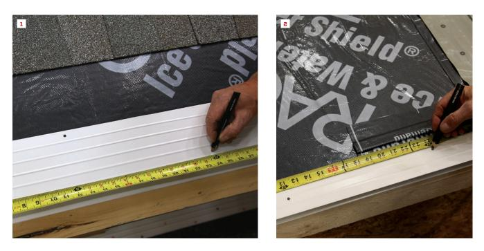
**Code requirements for nailing drip edge.** Code requires that the drip edge extend at least 2 inches onto the roof from the fascia board (1). This drip edge extends much farther. Nailing along the eaves should be spaced at no more than 12 inches on-center. Nailing should also be 12 inches on-center for rake drip edge (2). In both of these examples, the installer arranges the fasteners in a W pattern to put the drip-edge attachment closer to the edge of the roof.
